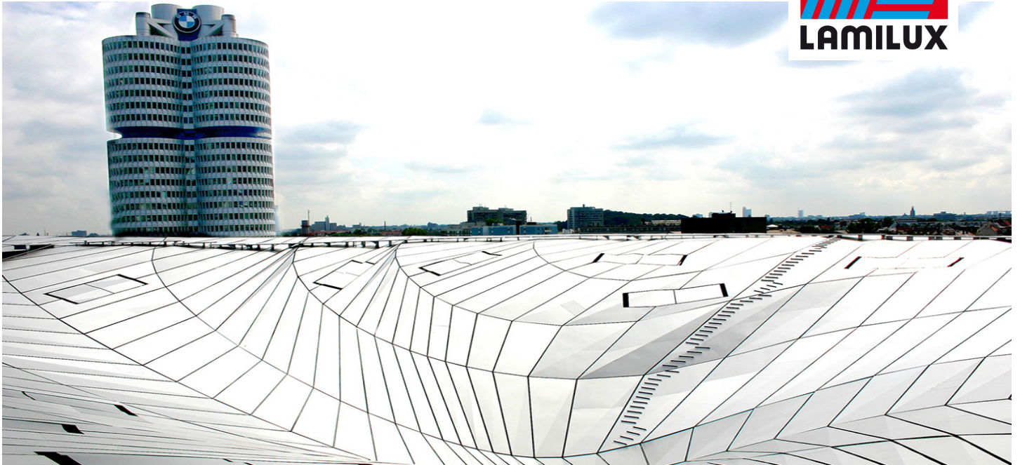
BMW Four Cylinder Building, Munich
